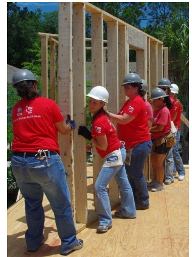
Lowe's employees and Women Builders frame a wall during National Women Build Week.
